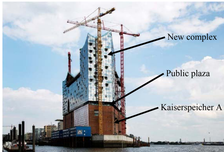
Figure 2: Construction site Elbphilharmonie (Thies Rätzke, May 2012)
