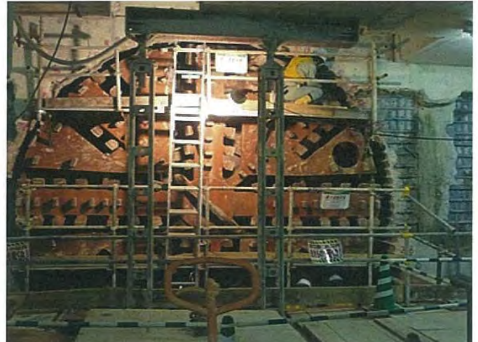
Photo-4 Arrival situation of the shield machine
