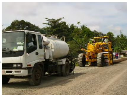
Photo-3 Mixing of cement and asphalt emulsion by PM550
