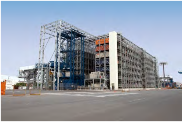
Photo – 1 General view of container hangar
