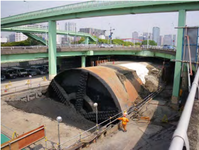
Photo-5 URUP Shield Arrival at Ground Level
