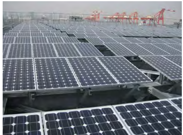
Photo – 4 Solar power generation system (generated output: 200kW)
