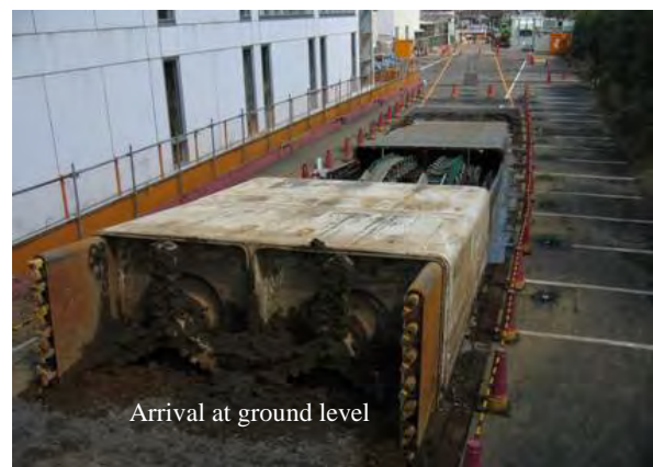
Photo-3 URUP Method Proving Test – Arrival
