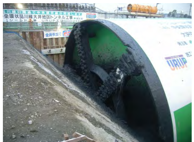
Photo-4 URUP Shield Launching from Ground Level
