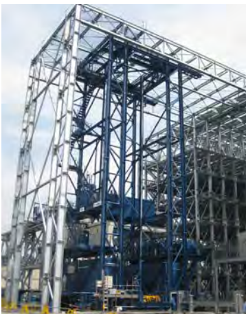
Photo – 3 Stacker crane
