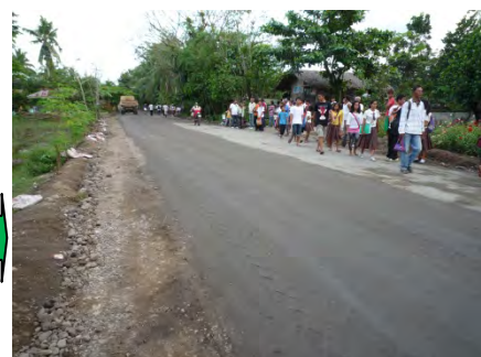
Photo-4 After surface finishing works
