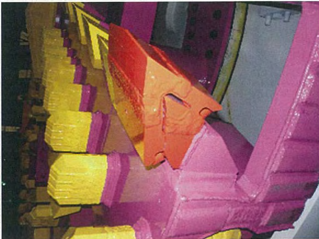
Photo-3 Installation situation of the double bit
